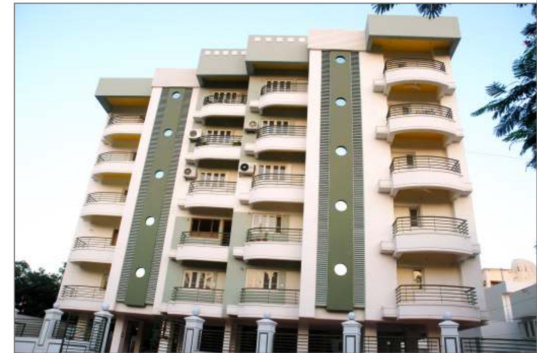
Neptune Tower - Sukhadia circle
